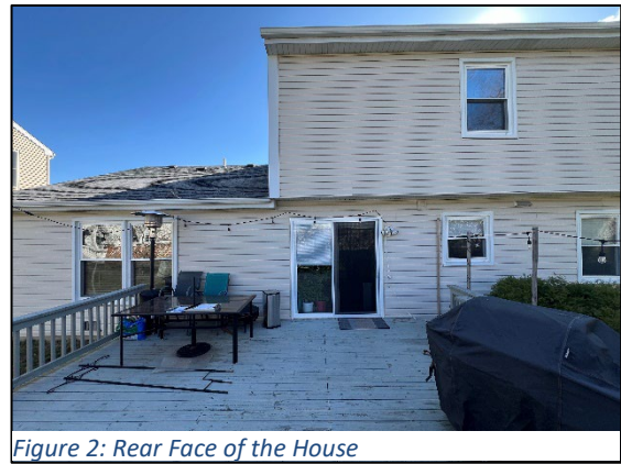
Figure 2: Rear Face of the House
