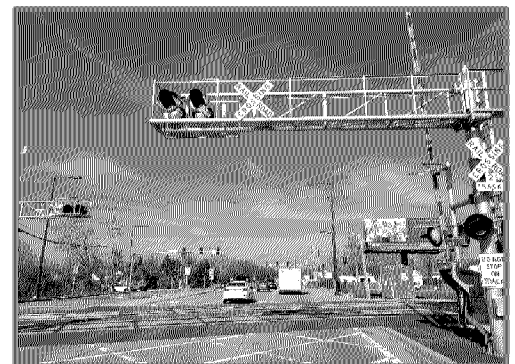
Looking west on IL 22, east of Prairie Rd./Main St.
