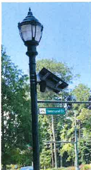
Solar & Existing Pole
