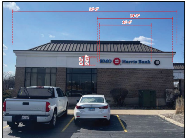
Figure 2: Existing Wall Sign on West Elevation
