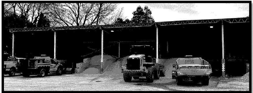
Storage Material Structures at Current Public Works Facility
