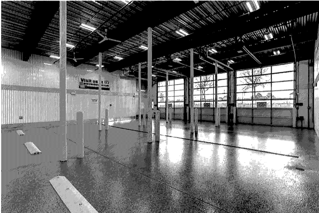
Metro Storage – Buffalo Grove IL – Loading Bays
