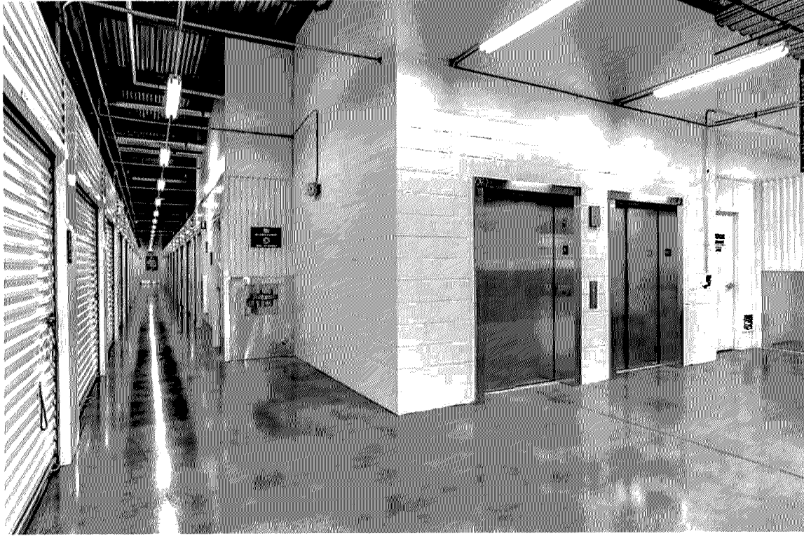
Metro Storage – Buffalo Grove IL – Elevator Bay and Typical Corridor
