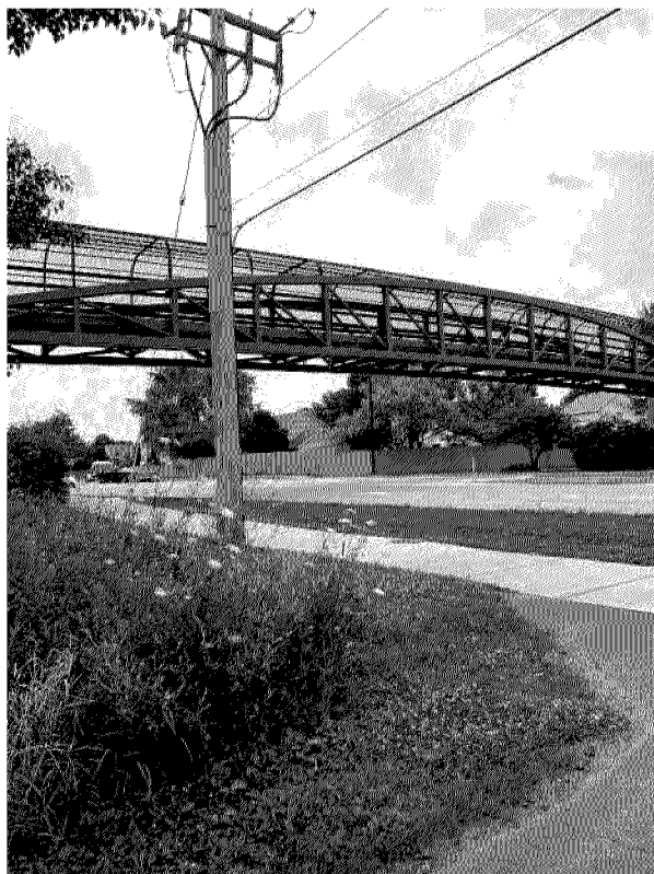
Southeast side of structure.
