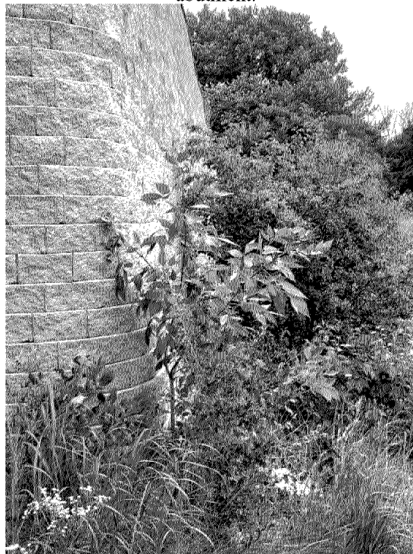
Significant woody plant growth along the northeast abutment.
