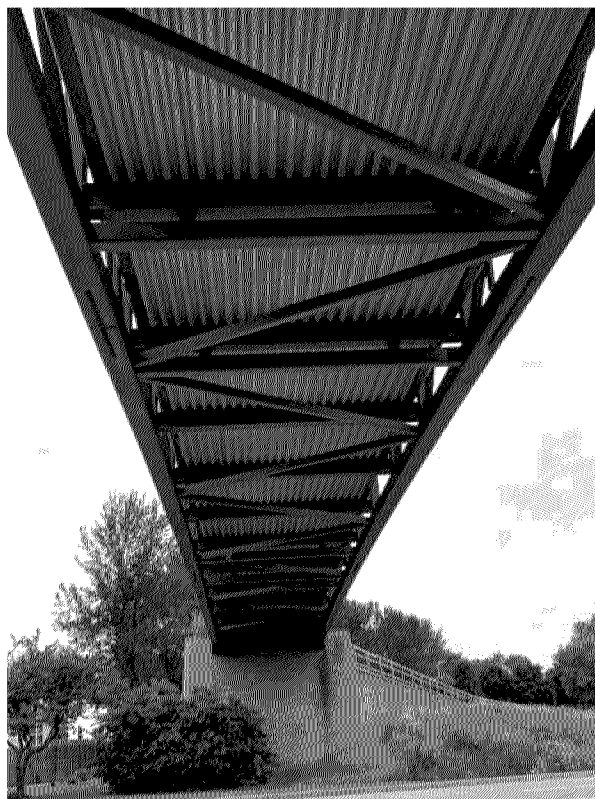
Underside of deck, looking northeast.
