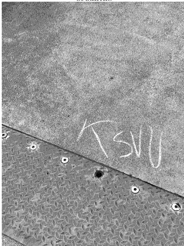
Bolt missing from the expansion joint covering plate.
