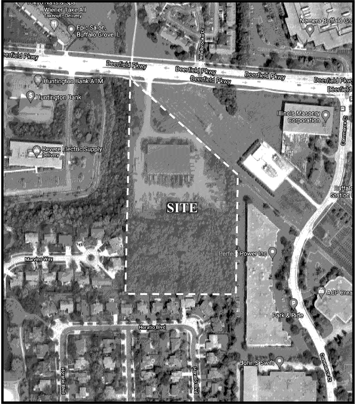
Aerial View of Site
