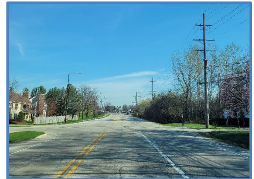
Looking north on Prairie Rd., south of Willow Pkwy
