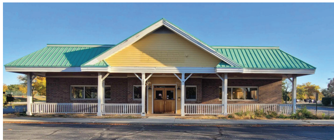
EXISTING BUILDING FRONT VIEW
