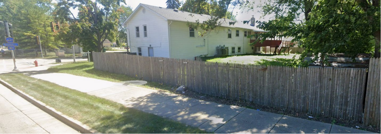
Figure 1: Existing Fence (Source: Google Street View)
