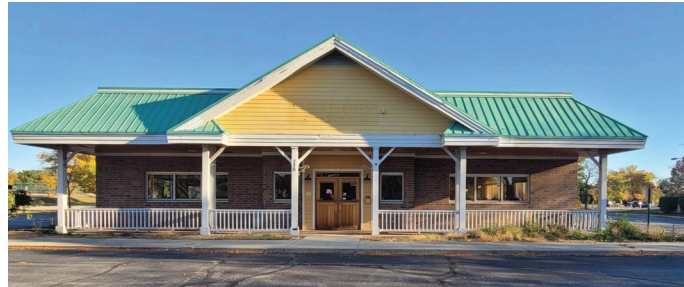
EXISTING BUILDING FRONT VIEW
