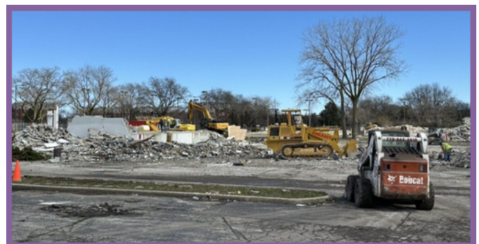
Spring, 2024 Demolition at the Bison Crossing Site
