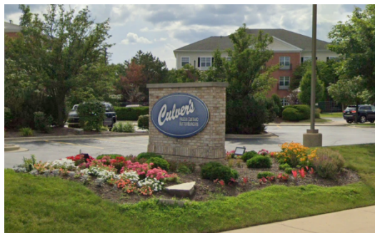
Figure 3: Existing Ground Sign with landscaping
